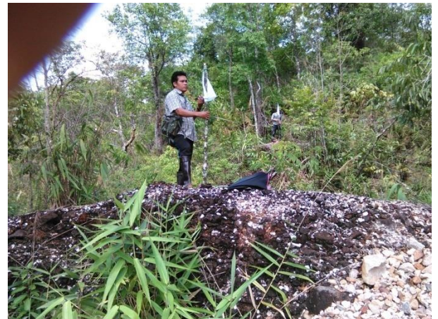
Final Tailing Pond (2)
